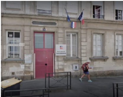
Nursery School Parcheminerie (France)
