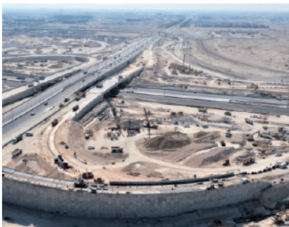
Al Khor Expressway (Qatar)
