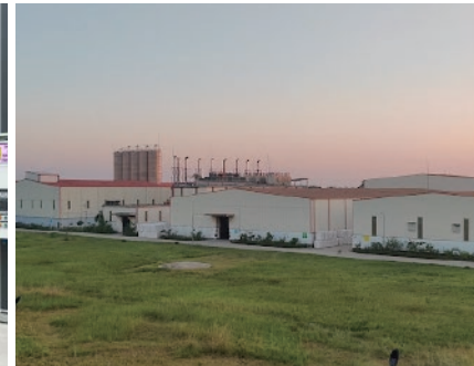
Akij Plastics Chhatak Plant (Bangladesh)
